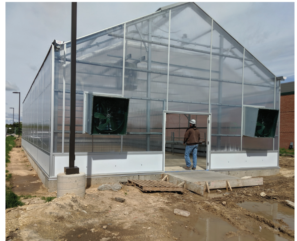
Completion of the Greenhouse
