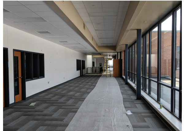
Second Floor Corridor in the Addition
