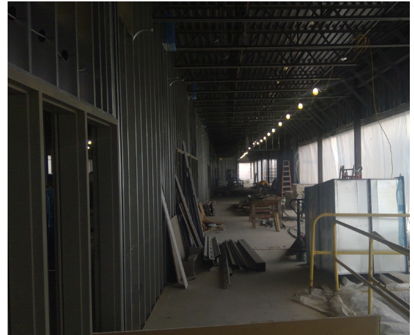
Wall Framing at Second Floor Corridor
