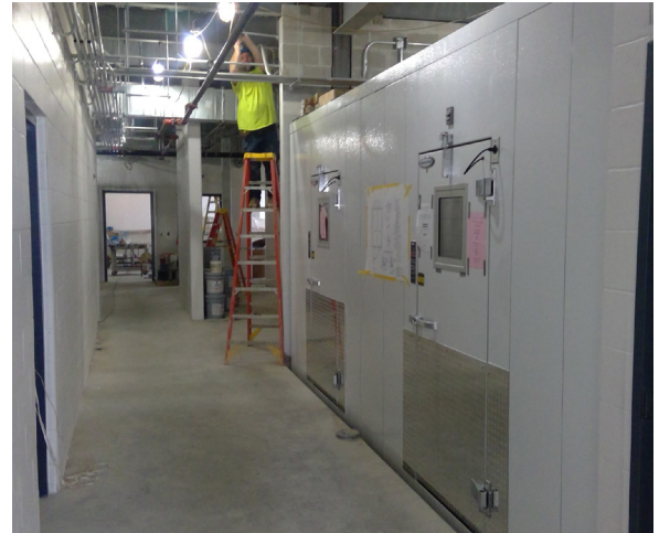
Equipment Installation in the Kitchen
