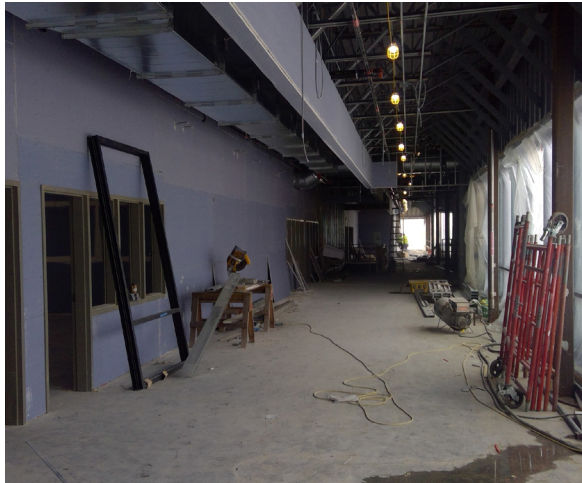
Drywall Installation in Second Floor Corridor
