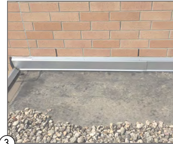
1 ROOF EDGE WITH METAL COPING
