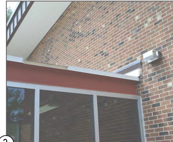
3 ROOF TO WALL CONNECTION WITH SCUPPER
