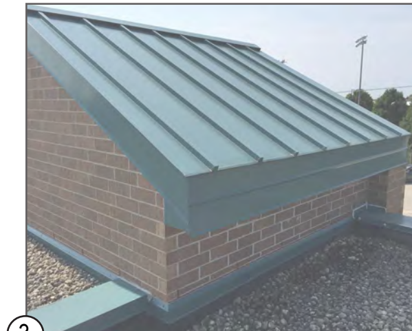
3 STANDING SEAM ROOF WITH SHEET DRAIN
