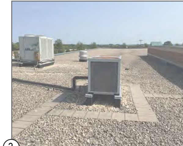
③ ROOFTOP MECHANICAL UNIT
