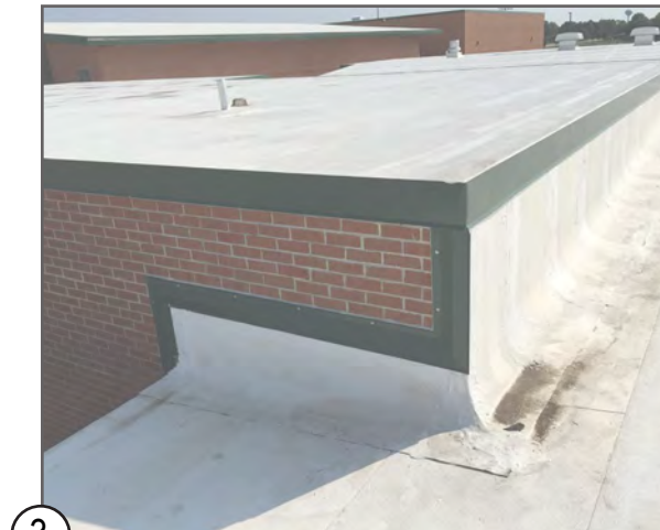
3 ROOF TO WALL CORNER CONNECTION
