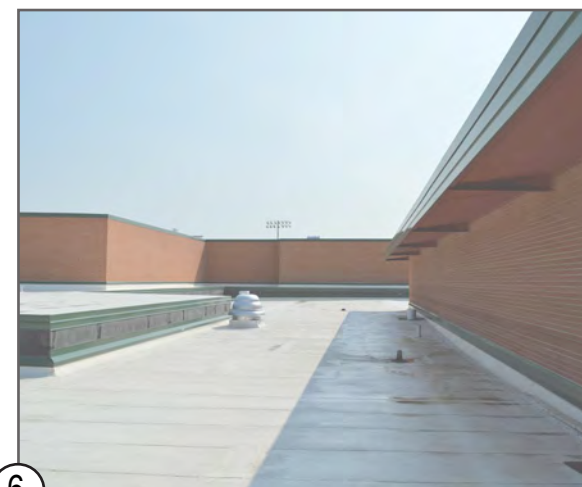
6 ROOF SOFFIT AND MULTIPLE ROOF TRANSITIONS
