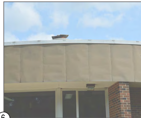
6 CIRCULAR ROOF METAL FASCIA
