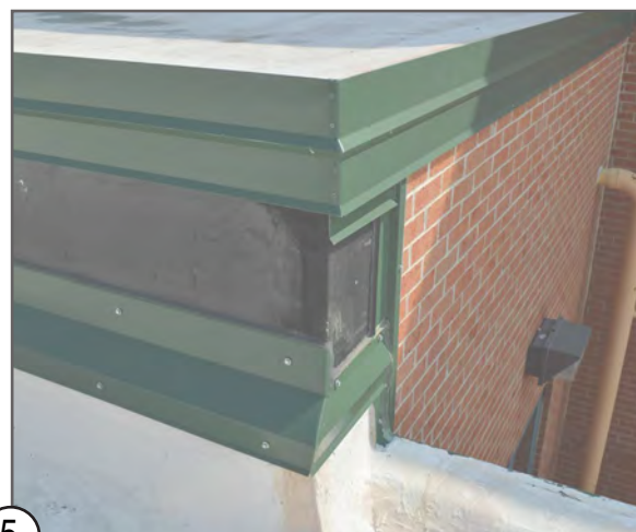
5 ROOF TO WALL CORNER CONNECTION
