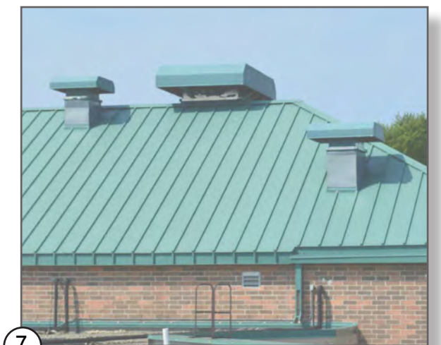
⑦ ROOFTOP VENTS
